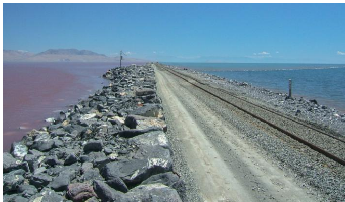
Figure 8. The railway causeway across the Great Salt Lake has caused major changes in the salinities on the two sides. Bridge and culvert construction continues to modify those salinity levels. Photo by W. Wurtsbaugh
